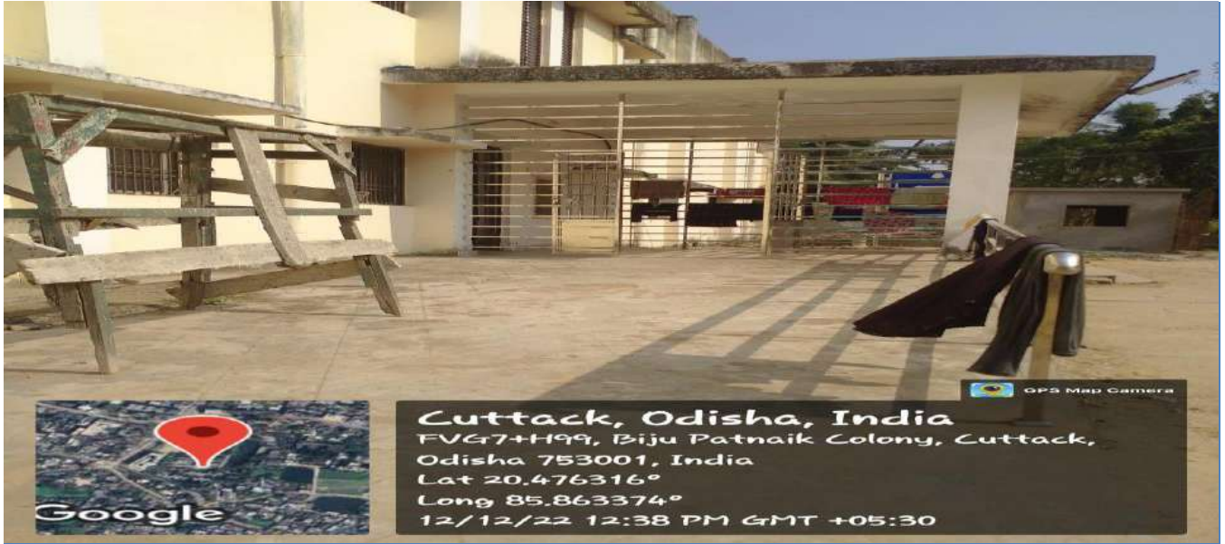
Ramp for Divyangjan
