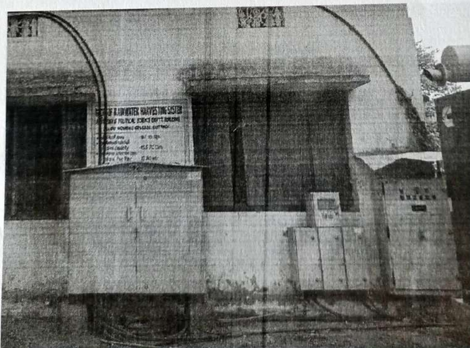
Roof top Rainwater Harvesting System installed in the College Campus
